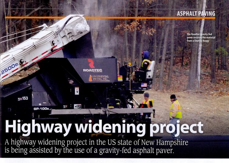
he widening work is being carried out as part of an upgrade for a 32km stretch of I-93, which was started eight years ago. The work is being carried out for the New Hampshire Department of Transportation (NHDOT) on a section of the highway between Exits 1 and 5 from the Massachusetts Stateline to Manchester, NH.
